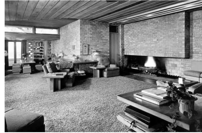
Lloyd Lewis House, Living Area Looking Toward Fireplace, Libertyville, Illinois, 1940, photograph
